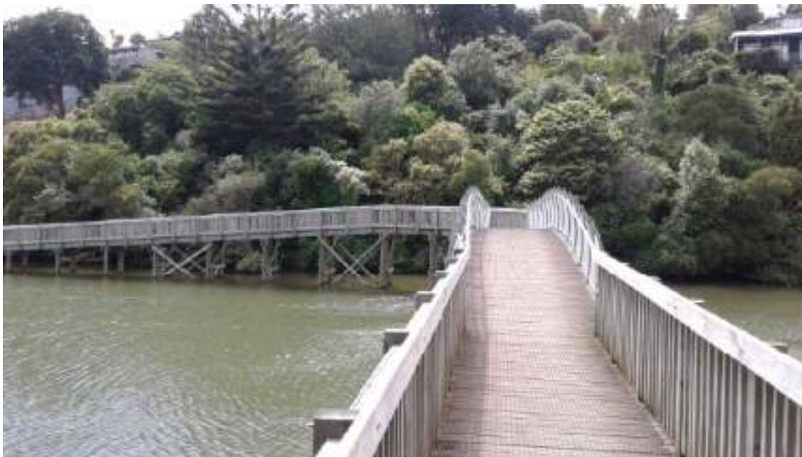
Figure 16: Pedestrian bridge across Ōrākei Creek
