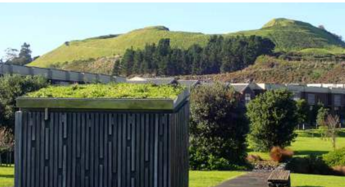
Roof garden in Stonefields. Photo by Kerry Lukies.
